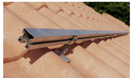
The hammer-head screw is now engaged in the mounting profile. Tighten the lock nut into the hammer-head screw of the **outermost** roof hook, so that the profile can no longer rotate or slip free from the roof hook.
